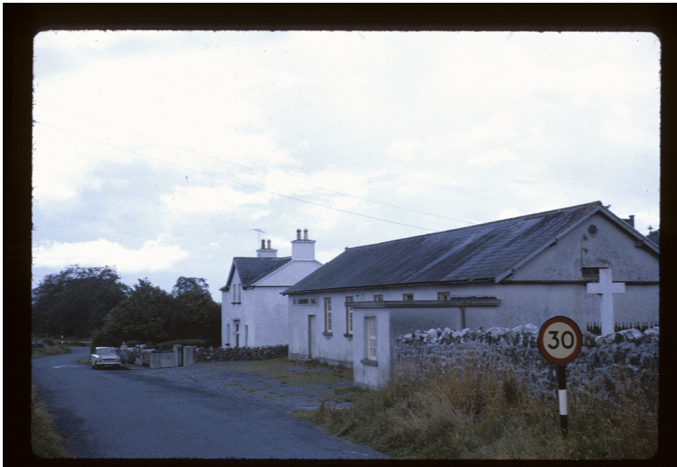
Fitzgerald House, The School and corner of the cemetery Aughrim
